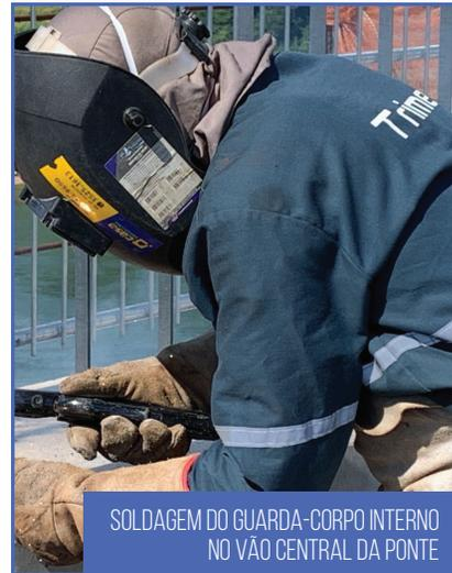
SOLDAGEM DO GUARDA-CORPO INTERNO NO VÃO CENTRAL DA PONTE
