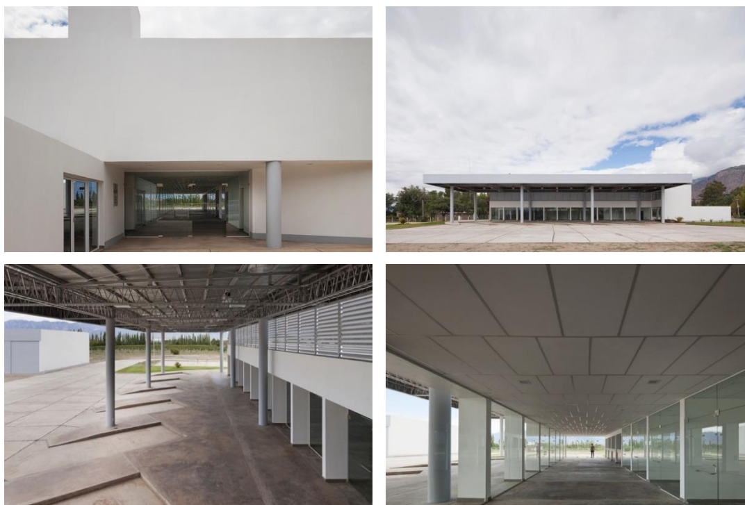
Figura 12 – Terminal de Cafayate (CCFGM)
